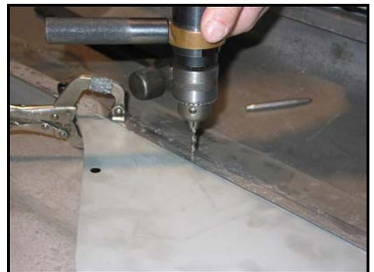
15. Repeat this process every 3" until the entire front and rear patch panel seams are attached.
