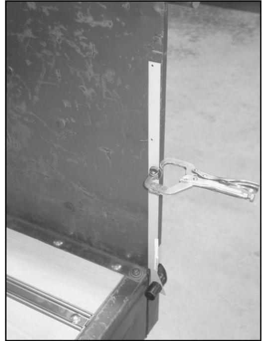
6. Mark the bedside through the two small 1/8" diameter holes in the template. These will be the location for the latch striker and the upper link mounting position.
