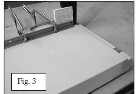
When you have the proper relationship between the angle strip and the rear sill and front bed panel, the angle is ready to install. Check that the front of the angle strip is toward the front of the bed and that it is exactly straight as clamped to the bedside. Be sure the bolt hole in the rear sill lines up with the rearmost angle strip bolt hole and that the bed strip holes line up with the angle strip holes.
