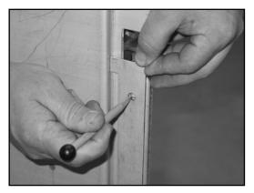
4. Remove the template and center-punch this location. Drill a 5/16" hole through the bedside at that location. Do this for both bedsides and deburr the drilled holes.
