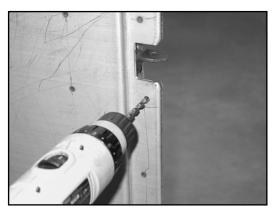
5. Install the fixed pivot pin into each of the 5/16 holes drilled in step 4. Use the 5/16" diameter button head screw to attach each pivot pin. Place the stainless washer over the fixed pivot pin before bolting it to the bedside. The screw head is on the outside of the bedside and the fixed pivot pin is on the inside of the bedside. Tighten the fixed pivot pin so that its flat edges are horizontal as shown in the photo.
