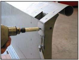
19. Remove the burr from the holes and install the supplied rubber grommets.
