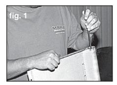
2. Insert the tie rod end without hardware through the top hole in bed side. Secure with a 5/16" flat washer, lock washer, and nut. Bolt the front bed panel side flange to the inside of the bed side with (4) 1/4"-20 x 5/8" hex head bolts, lock washers, and nuts. See figure 2.
