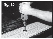
22. Using a 1-9/16" diameter Forstner bit, a drill press if available, or a hand drill, countersink each location approximately 1/8" to 5/32" deep. See figure 15.
