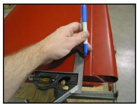
4. Measure towards the bottom of the tailgate from this line 2-5/8" and make another mark. Make a 1-7/8" line on this mark as before. Join the ends of these two lines to create a rectangle
