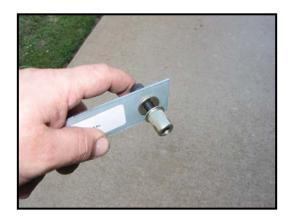
12. Place the insert into the hole in the bed side. Make sure to hold the insert flange tight against the bed side. This scrap metal will act as a handle to keep the insert from rotating when the nut is tightened. It would be beneficial to have a helper for this step to hold the scrap metal handle.
