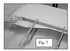
2. Remove the angle strip and draw a line the length of the bedside at the position of the plug welds, about 3/8" above the bottom of the angle strip. The welds should be midway between the bottom leg of the angle and the rolled edge of the top of the angle. See figure 8.
