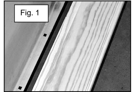
9. Mark all holes through the bed side lower lip onto the wood boards. See figure 2. Remove these two boards and drill each location through with a 3/8" wood bit. See figure 3. Back up the boards with a piece of scrap wood to keep the boards from splintering on the bottom side.
