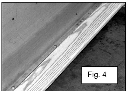
14. The next two boards to be installed on each side are 9-1/8" wide overall. Place these boards next to the outer boards but leave a 1/2" gap between them and the outer boards. Again make sure they are grooved side up.
