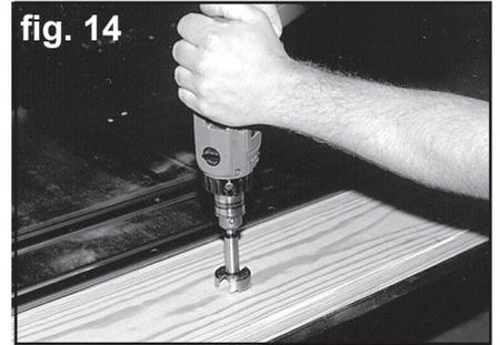
23. Using a 1-9/16" diameter Forstner bit, a drill press if available, or a hand drill, countersink each location approximately 1/8" to 5/32" deep. See figure 14.
