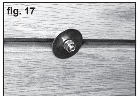
28. Where there is not a cross sill or reinforcement strip under the bed strip holes, install a 1-1/2" outside diameter washer with a 1/4" diameter hole before installing lock washers and nuts. See figure 17.
