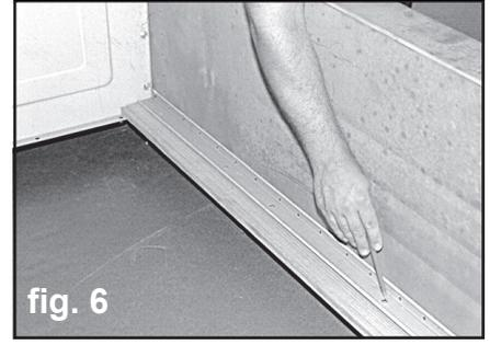
9. Mark all holes to be drilled in the edge boards through the angle strips holes. See figure 6.
